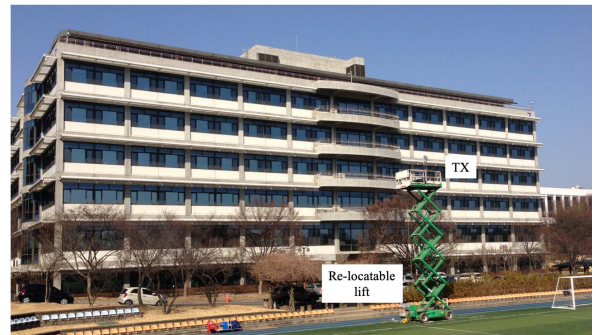
(a) Building A
