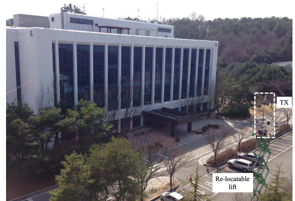
(b) Building B
